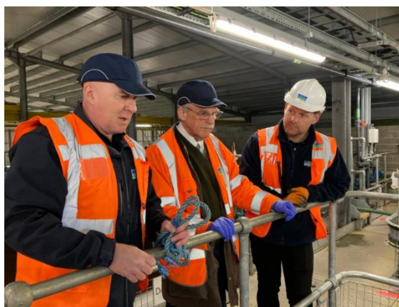
Mark Isherwood, MS for North Wales, visits Llwyn Onn Water Treatment Works
