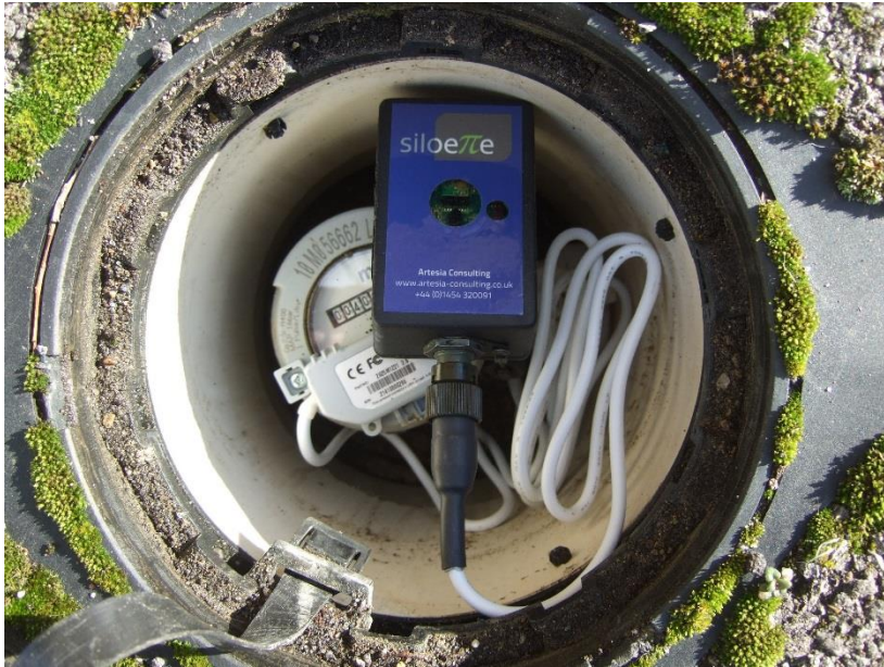
Figure B2.14 Siloette logger installed in a boundary box
